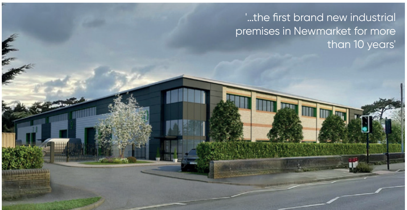
Nucleus Business Park, Newmarket, now under construction
