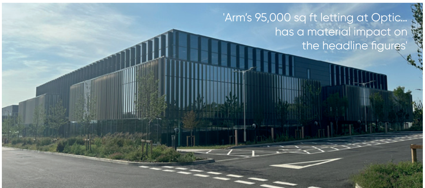
Optic, Peterhouse Technology Park
